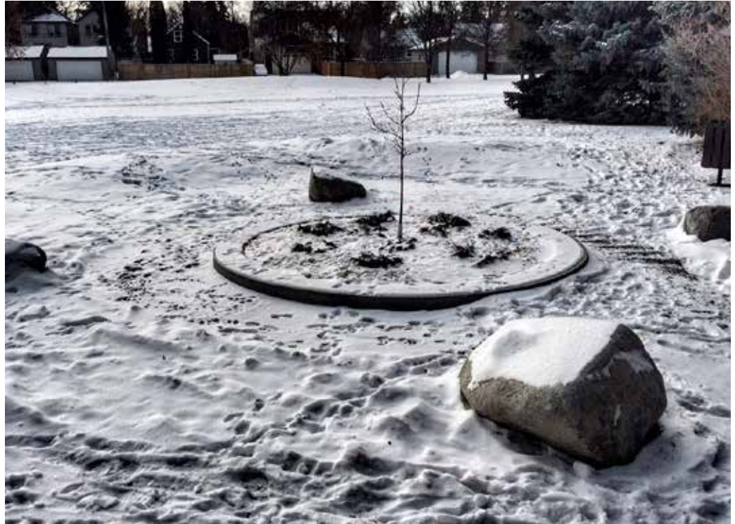
Raoul Wallenberg park, as of last month. Contractor Mark Bobyn made good use of the beautiful October weather and managed to complete the project before the snow fell. Only the new sod will need to be watered in the spring.
